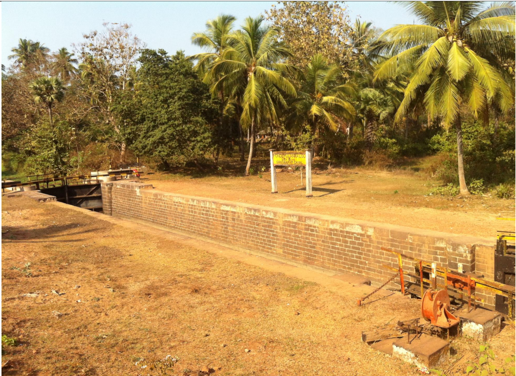
The masonry of these locks, older than our Freycinet locks, is in an astonishing state of conservation, but it must be said that there has been practically no navigation for 30 years.
